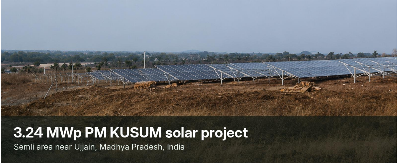
Figure 1. Constructed solar array for the 3.24 MWp PM KUSUM project near Ujjain, Madhya Pradesh, India.
